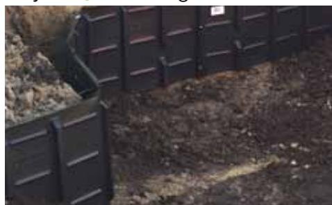
RootBarrier® RootPanels® Rib wortelgeleiding
